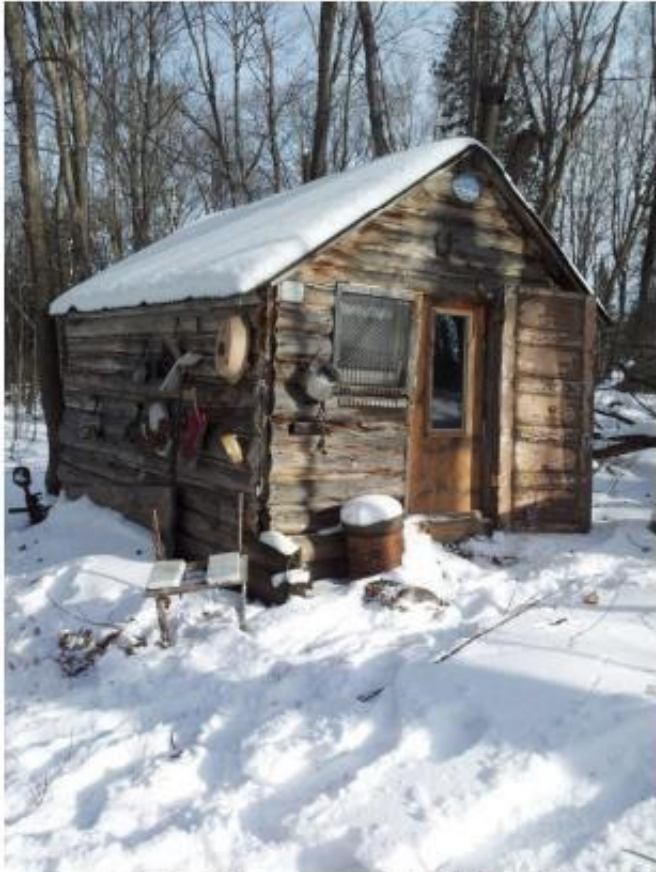
Algoma District, camp built in the 60's, the logs were cut in half so that one half of the log would make one wall the other half would make the opposite wall.
